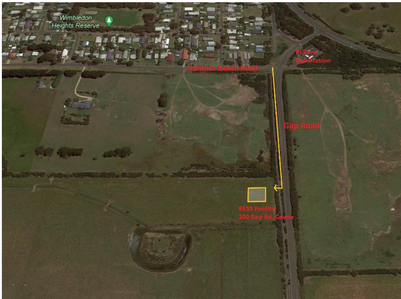
Figure 5: Phillip Island Community Battery on Gap Rd in Cowes 4
